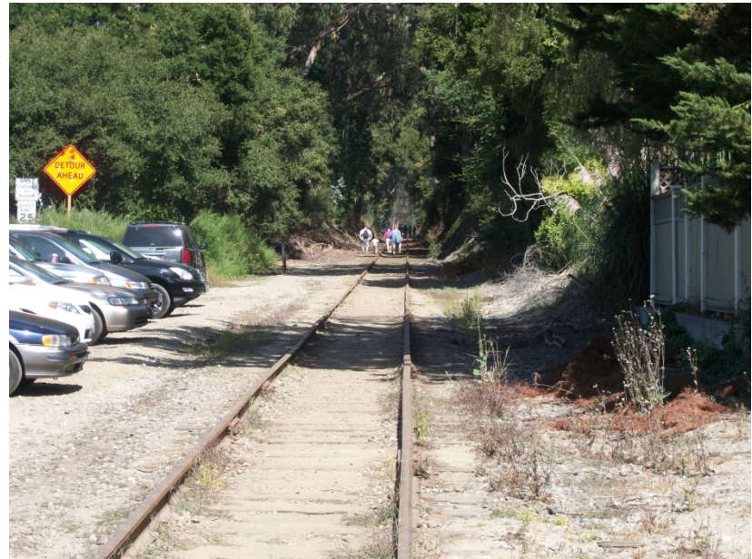
Santa Cruz Branch Line right-of-way
