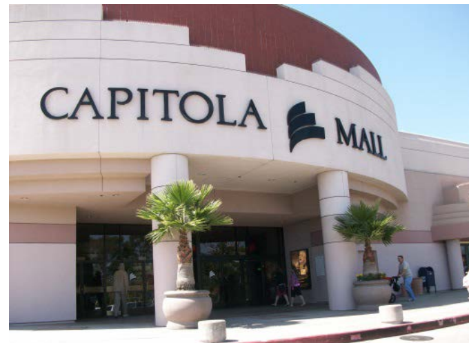
Best Western hotel (top) and Capitola Mall (bottom) on the 41 st Avenue corridor.
