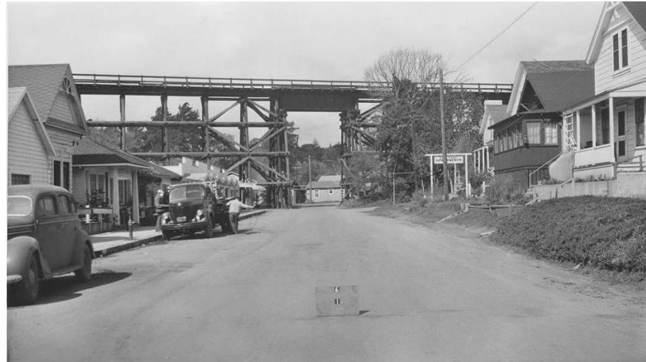
Historic trestle crossing Capitola Avenue
