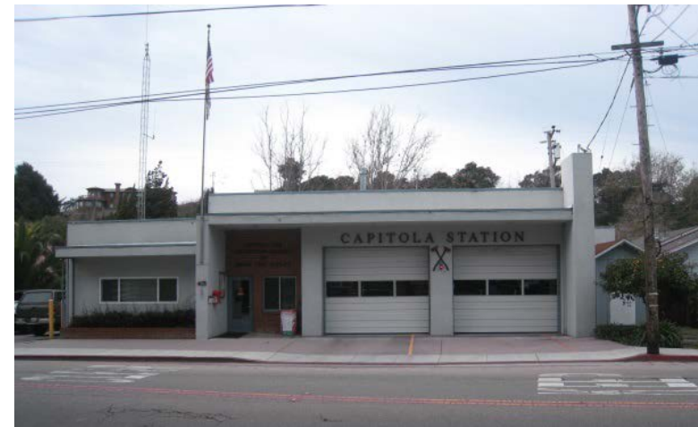
Property on bluffs impacted by erosion and landslides (top) and CFPD fire station on Capitola Avenue (bottom)
