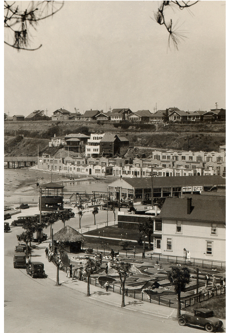
The Esplanade, Venetian, and Cliff Drive homes
