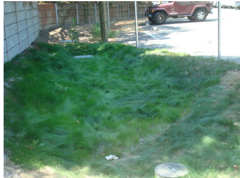
Stormwater bioretention swale
