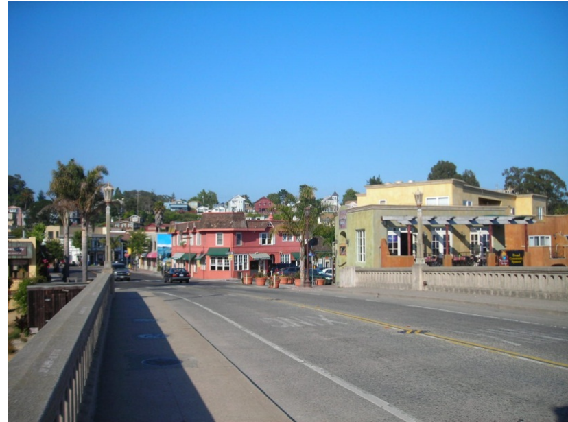
Stockton Bridge crossing Soquel Creek
