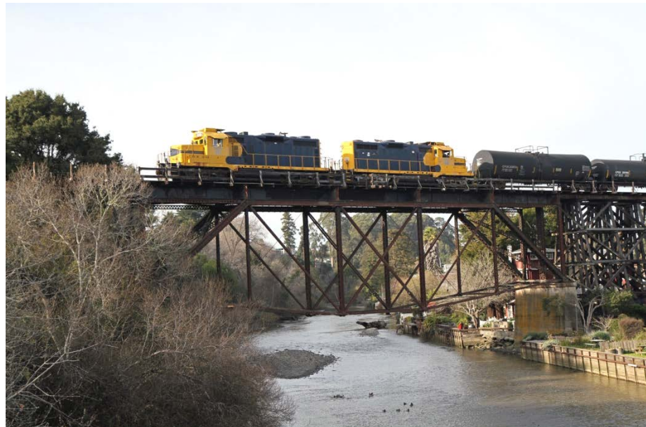
Freight rail service crossing the trestle
