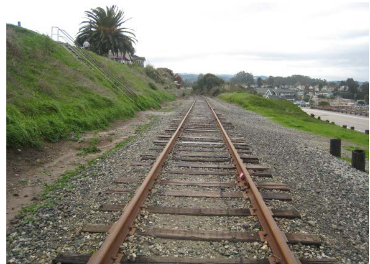
Railroad right-of-way along Cliff Drive
